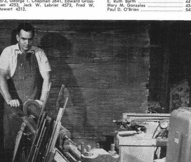
PATIENCE is a virtue in hand-boring muzzle-loading rifles. Dick Hicks uses boring machine he built to Colonial period specifications.
